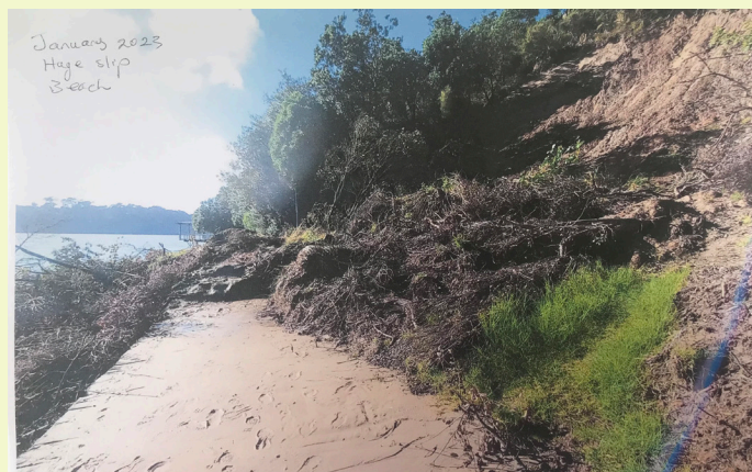
Initial slip at Blockhouse Bay Beach January 2023. This was followed by further erosion and slippage during subsequent weather deluges that lasted until early March. The walkway was cleared twice during this time. The debris of mud and broken trees remains to this day in the water below and at the base of the slope.
