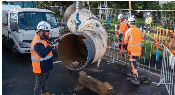
Above: Old Huia watermain pipe being lifted out of Heaphy St
